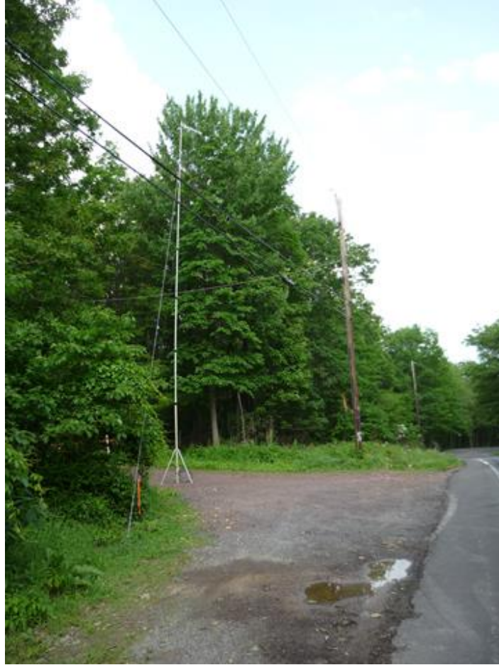
Figure 4: 2011 Weatherly B TLink Antenna Mast
