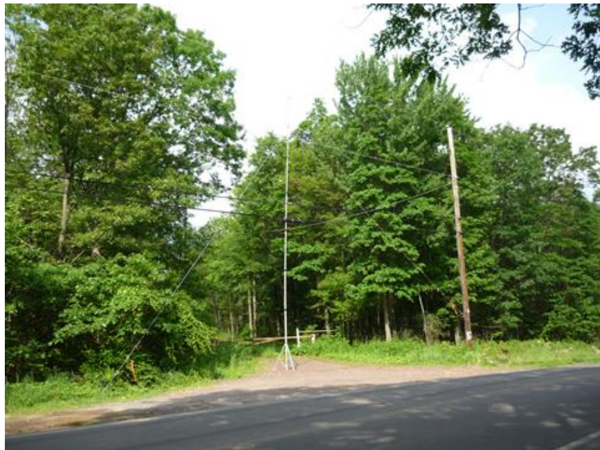
Figure 5: 2011 Weatherly B TLink Mast Base and Guy Lines
