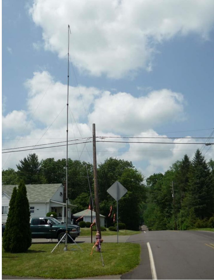
Figure 2: Weatherly Z TLink Antenna Mast
