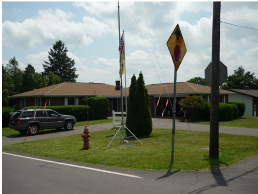
Figure 3: Weatherly Z TLink Mast Base and Guy Lines
