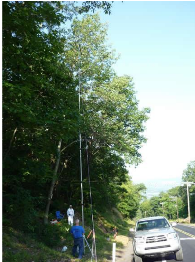
Figure 5: Giants Despair B T-Link Antenna Mast Direction
