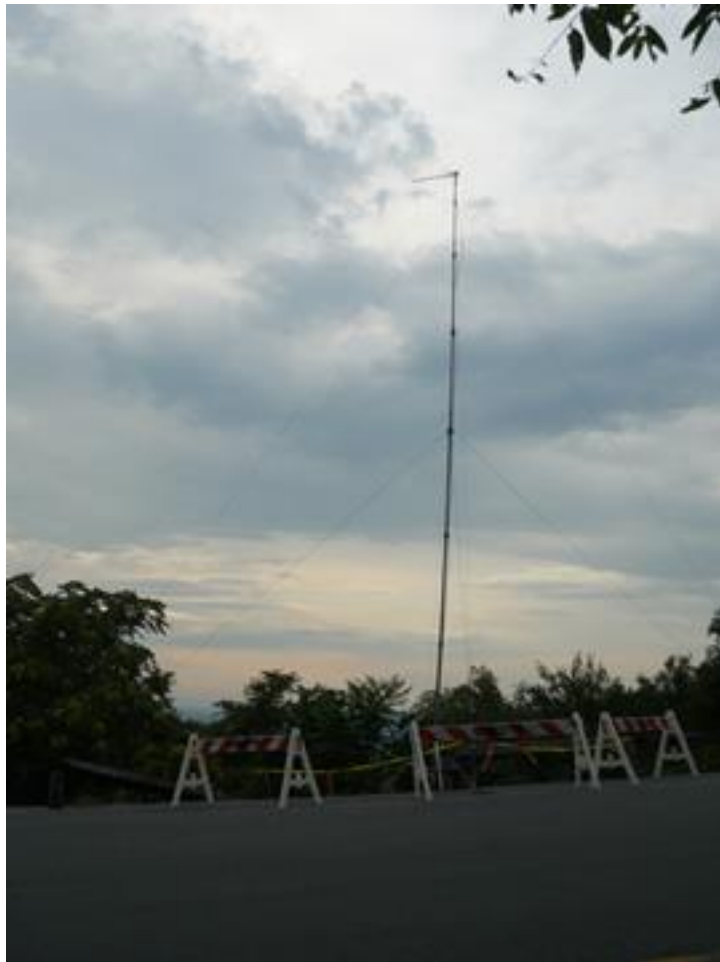
Figure 5: Duryea B T-Link Antenna Mast Base Location
