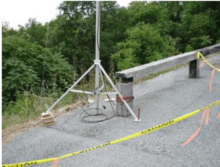
Figure 4: Duryea B T-Link Antenna Mast Base Position
