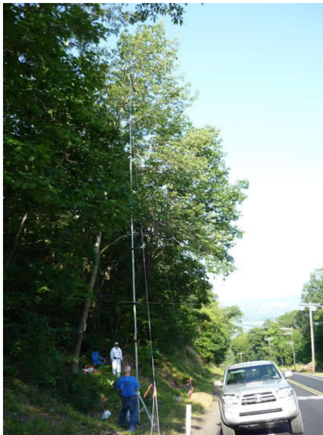
Figure 5: Giants Despair B T-Link Antenna Mast Direction
