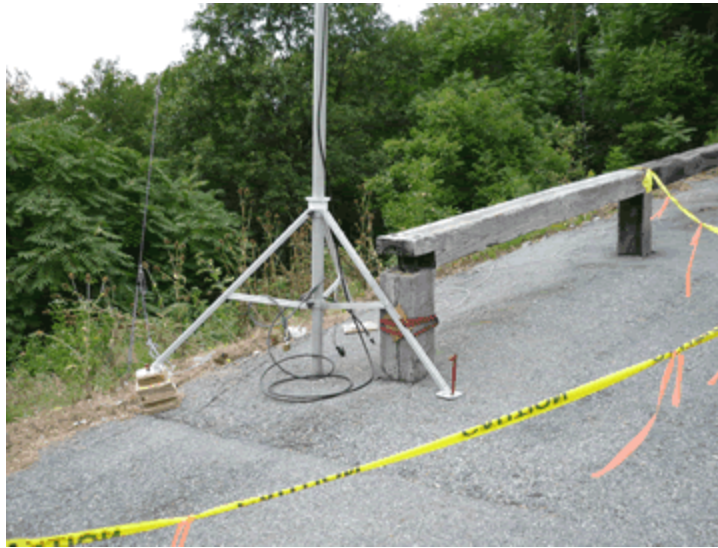
Figure 4: Duryea B T-Link Antenna Mast Base Position
