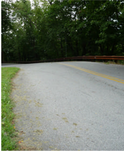
Figure 6: Duryea A T-Link Antenna Mast Location
